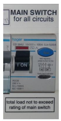
If a fault occurs, or a person gets an electric shock, a small amount of current flows from Live to Earth – this is the residual current. The current in the Neutral wire is less than the current in the Live wire. A Residual Current Circuit Breaker (RCCB) detects the small difference in current in the Live and Neutral and disconnects the electrical supply. An RCCB is very fast, disconnecting the supply in just a few milliseconds.
