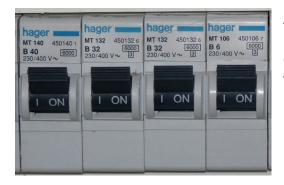
A circuit breaker does the same job as a fuse, it breaks the circuit if too much current flows. A circuit breaker is an electro-mechanical device which means it uses an electromagnet to move a mechanical switch when the current is too high.
