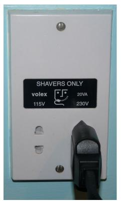
Isolating transformerTransformers are used to convert a high a.c. voltage to a lower, safer a.c. voltage.
